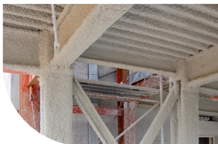
ST. THERESA VILLA - BAGHERIA (PA) - ITALY
