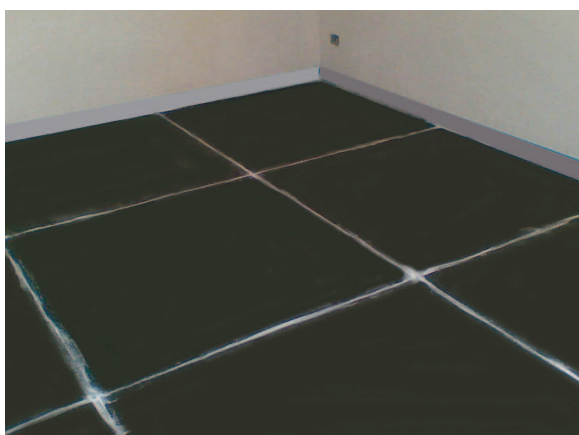
3. dBred mat applied in a continuous way with AD series perimetric stripes
