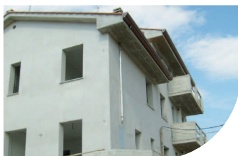
External wall insulation (EWI)
