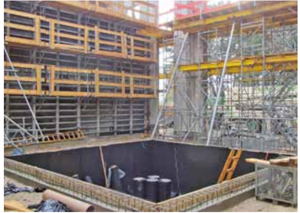
Flight simulator Airbus A400M, Wunstorf, Germany: full-surface decoupling of machine foundation with Regupol®
