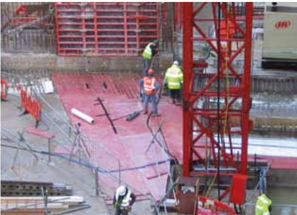
Southampton Row, London, UK: full surface decoupling of the building foundation with Regufoam®
