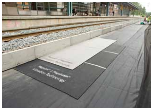
Commuter train station, Helsinki, Finland: Regupol® ballast mats
