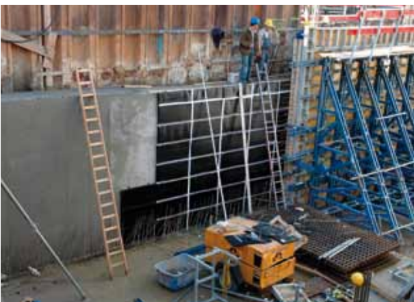
Kurfürstenplatz, Munich, Germany: vertical decoupling of the building foundation with Regupol®
