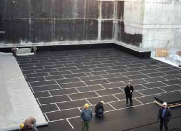
AGBU administration building, Jerewan, Armenia: full-surface decoupling of the building foundation with Regupol®
