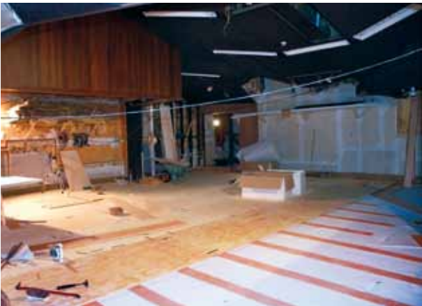
Wisselord-Studios, Hilversum, Netherlands: room-in-room construction with Regufoam ®
