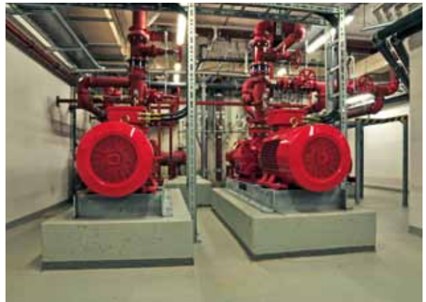
Nextower, Palaisquartier, Frankfurt, Germany: vibration isolation of heating, ventilating, and air conditioning with Regupol®
