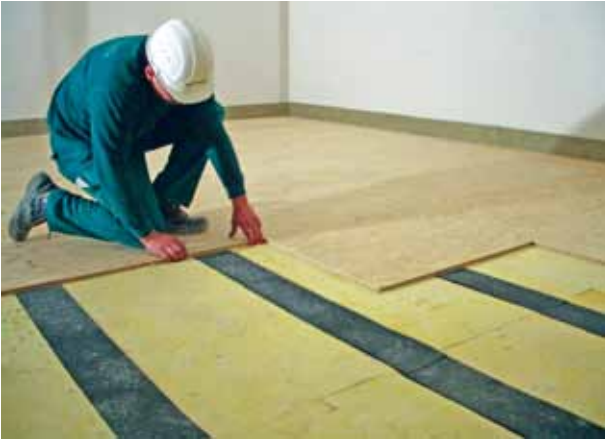
RTL-Studios, Cologne, Germany: room-in-room construction with Regupol ® impact sound insulation under screed
